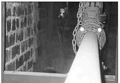
A dark inviting steam tunnel beneath Ohio State
